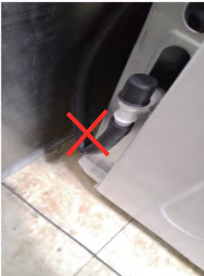
Drain hose connection incorrectly.
